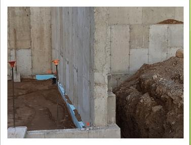
Compacted fill being added below North portion of gym floor
