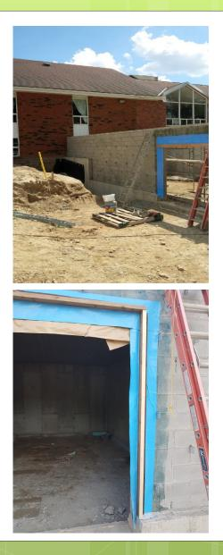
Exterior masonry walls completed at storage rooms below future kitchen and ready for precast concrete slabs.
