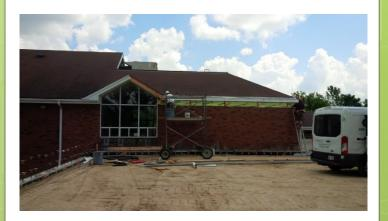
Les and Steve complete removal of soffit extension at existing wall and making it watertight in preparation for masonry wall construction
