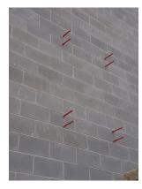
Masonry anchors installed in preparation for brick installation
