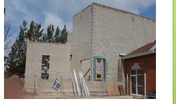
Masonry walls complete except at Platform and storage rooms
